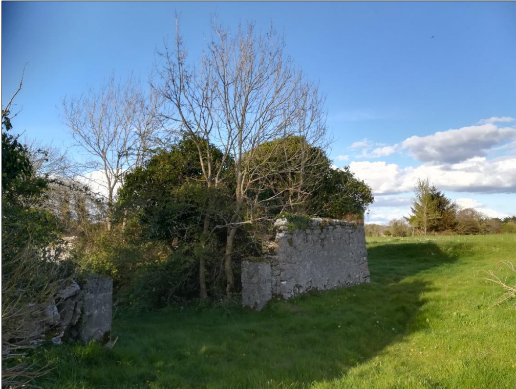
Plate 3-7: Buildings and artificial surfaces (BL3); silage pit constructed within the site of a habitat within stone walls (BL1) remaining from a building in ruin with areas of scrub (WS1) within the development site boundary.
