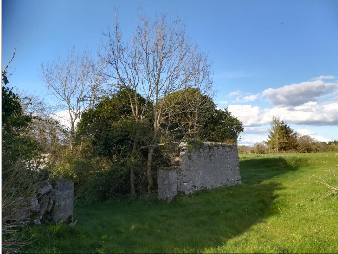
Plate 2.7 Buildings and artificial surfaces (BL3); silage pit constructed within the site of a habitat within stone walls (BL1) remaining from a building in ruin with areas of scrub (WS1) within the development site boundary.
